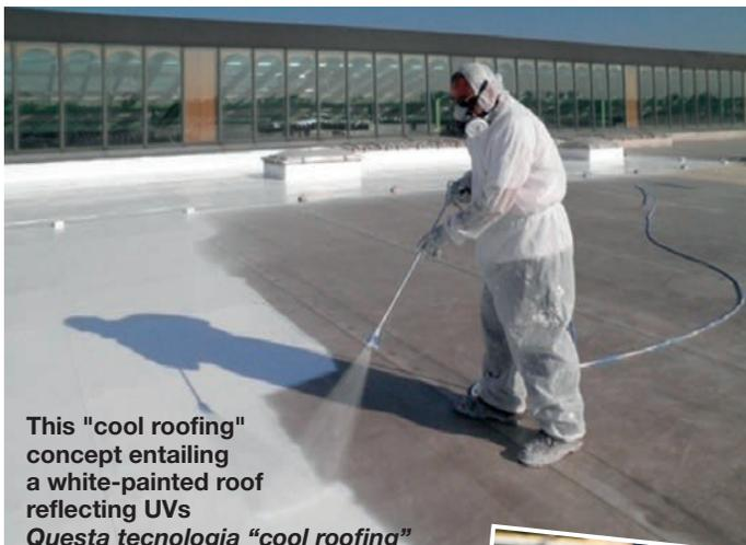
This "cool roofing" concept entailing a white-painted roof reflecting UVs
