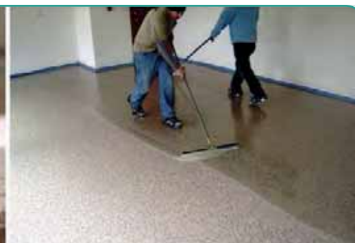
Fig. 9 IC-1 based topcoat applied by squeegee and single back-roll Finitura a base di IC-1 applicata a spatola e unica posa a rullo
