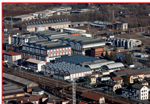
Overhead view of the Villadossola plant nowadays
